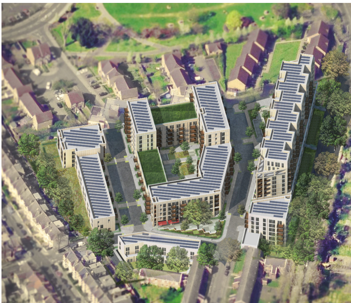
Aerial view of the new Sherwood Close
